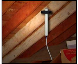
Figure 5 - Mounting Signal Antenna to a Main Beam
